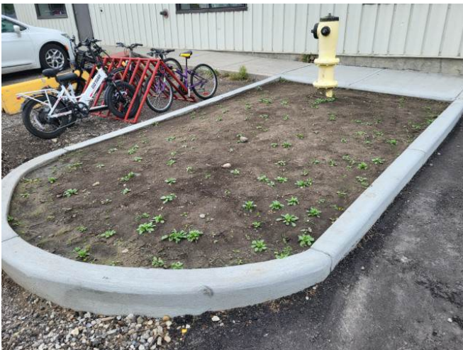
Aug 15_ Concrete Curb Constructed Around Fire Hydrant
