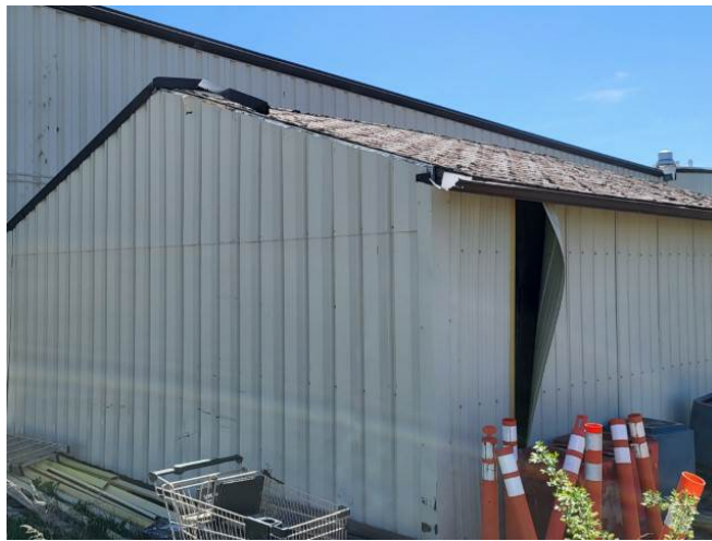
Photo #55: Storage Shed - Dislodged Wall Metal Cladding
