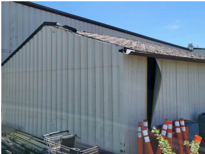
Storage Shed - Dislodged Wall Metal Cladding
