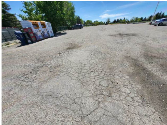
Photo #59: Deteriorated Parking Lot Asphalt Pavement
