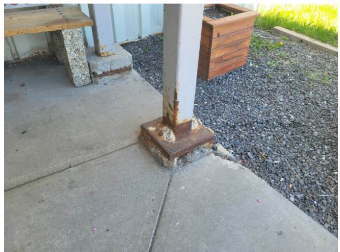
Corroded and Deteriorated Base of the Canopy Columns and the Columns Supports
