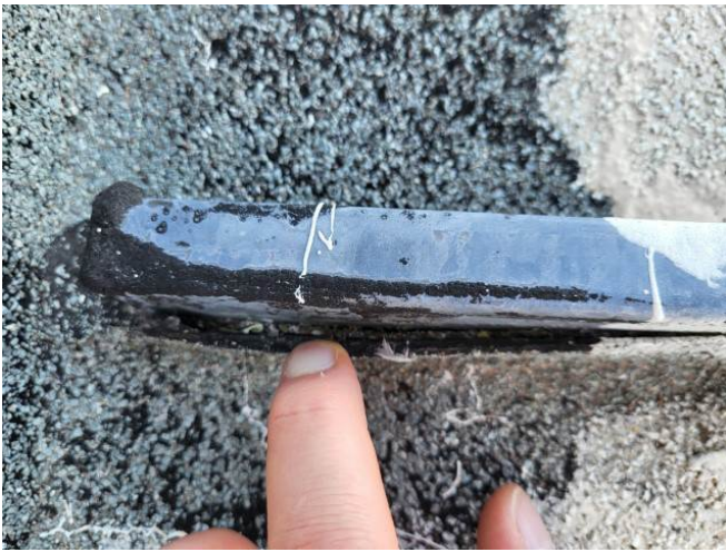
Debonded Roof Repairs Near Ribs
