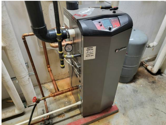
Photo #66: Boiler Serving the Snow Melt System
