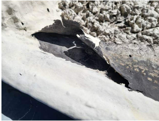
Photo #27: Debonded Roof Repairs
