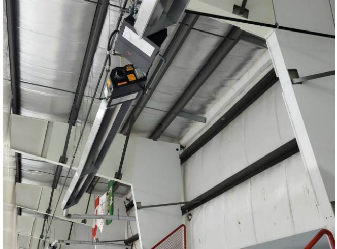
Suspended Infrared Heater
