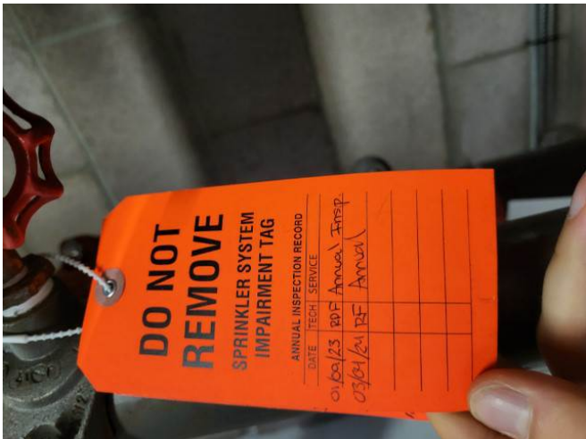
Sprinkler System - Overdue for Inspection
