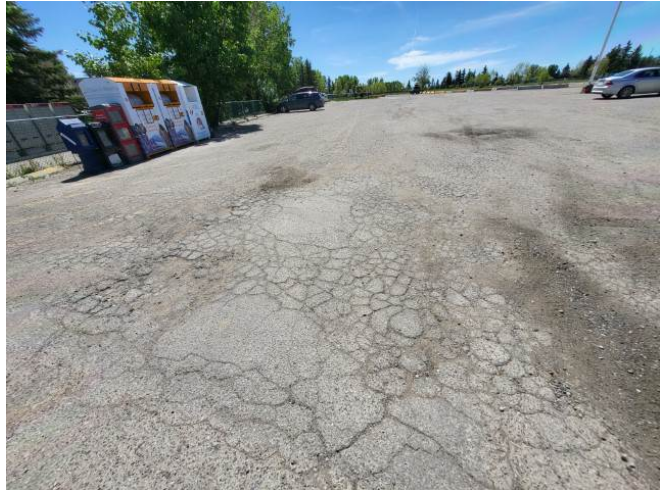
Deteriorated Parking Lot Asphalt Pavement
