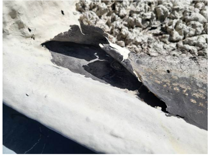
Debonded Roof Repairs
