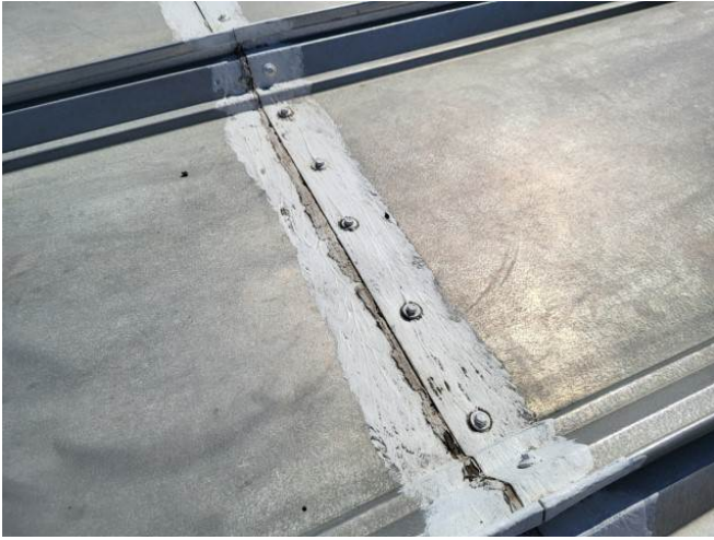
Deteriorated Roof Repairs - Fasteners
