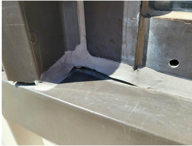
Photo #19: Debonded Perimeter Window Sealant
