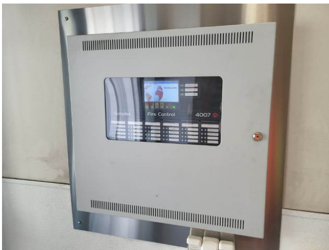
Fire Alarm Control Panel
