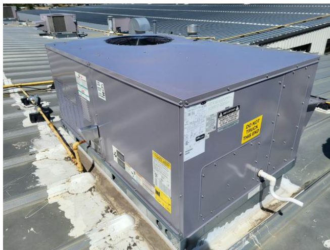
Photo #67: Typical RTU
