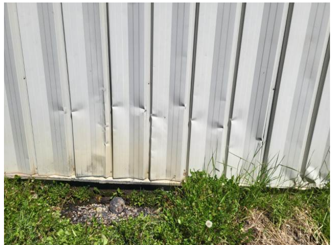
Dented Cladding - South Elevation
