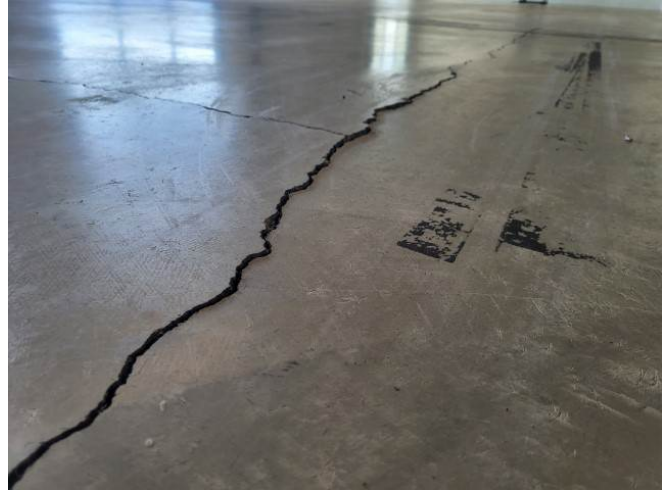
Cracking and Displacement in the 2nd Floor Slab of Undeveloped Area
