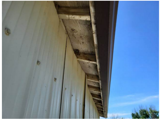
Storage Shed - Missing Overhangs Soffit
