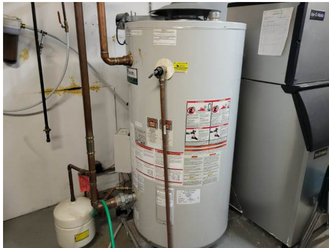
Photo #74: Domestic Hot Water Heater Serving Blue Arena
