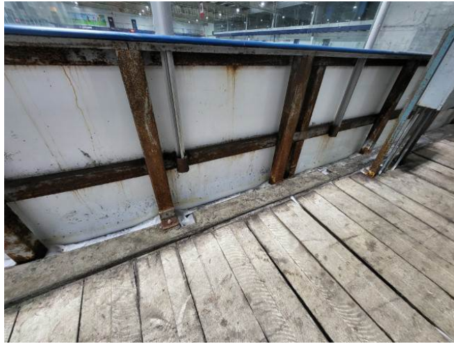
Photo #42: Corrosion on Dashboards - Blue Arena
