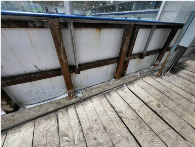
Corrosion on Dashboards - Blue Arena
