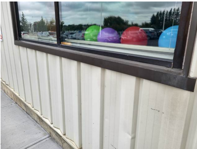
Aug 15 _Window Sill Sealant Replaced
