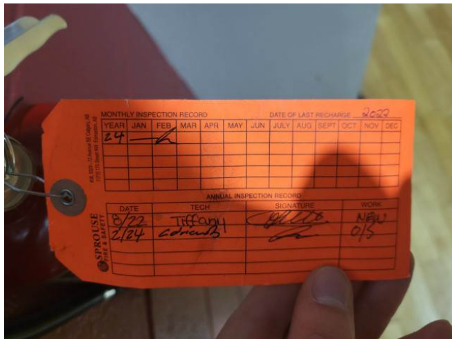
Photo #35: Fire Extinguishers - Overdue for Inspection
