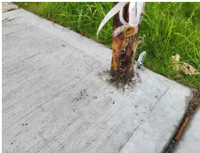
Photo #49: Aug 15_ Railing Imbedded in Concrete_ Corrossion Present
