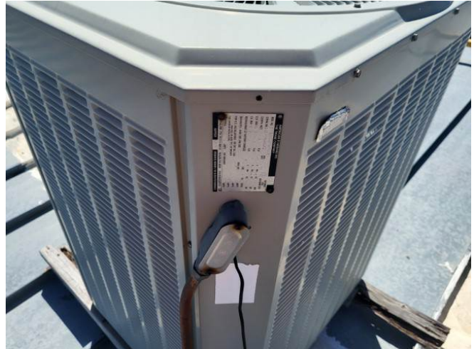
Condenser connected to Furnace
