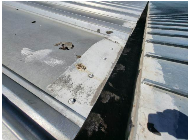
Roof Drain Trench
