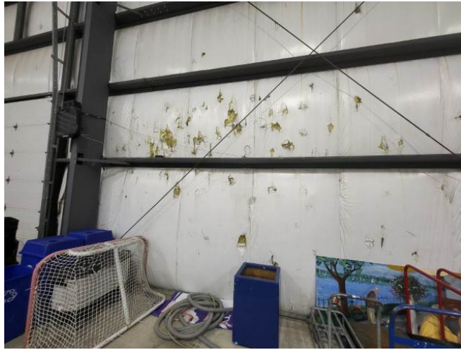
Photo #16: Damaged Insulation and Vapour Retarder on the Interior Face of Red Arena Walls
