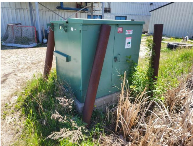
Pad Mounted Transformer - Tilted Bollards
