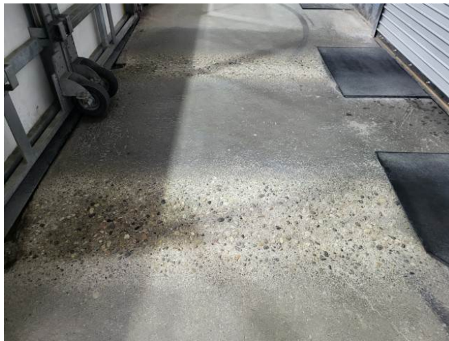
Photo #8: Deteriorated Slab on Grade in Zamboni Garage (Small)
