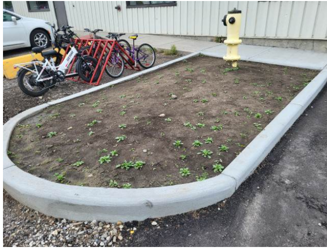
Photo #63: Aug 15_Concrete Curb Constructed Around Fire Hydrant
