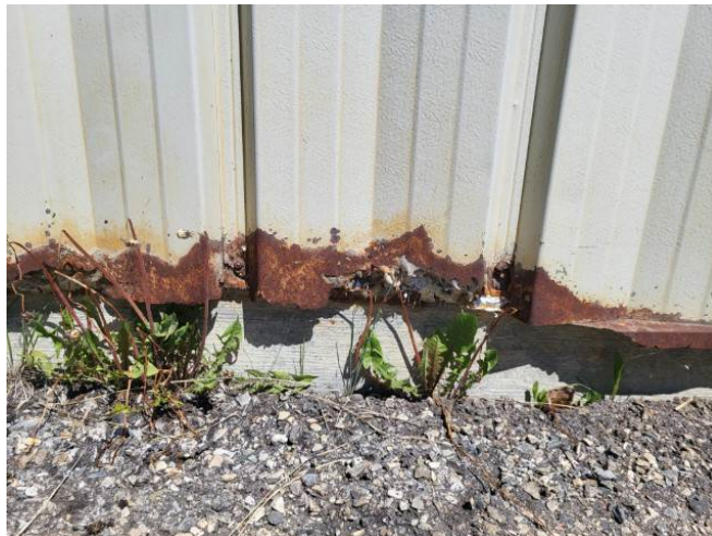
Photo #15: Corroded Metal Panel Cladding - South Elevation
