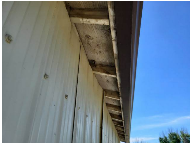
Photo #53: Storage Shed - Missing Overhangs Soffit
