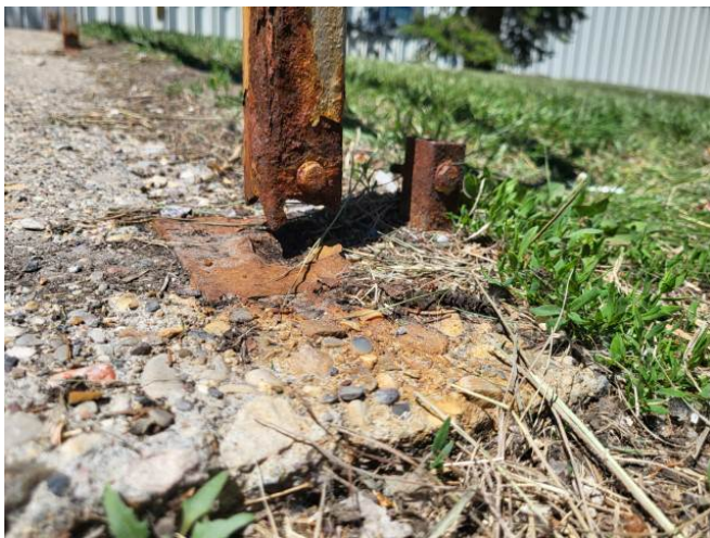
Corroded Railing - Entrance
