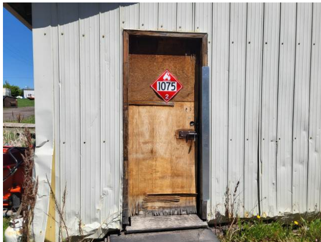
Photo #56: Storage Shed - Deteriorated Man Door
