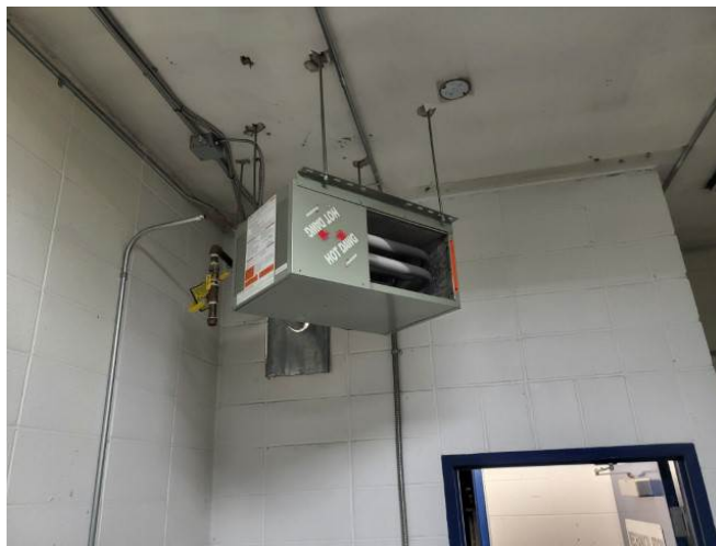
Photo #70: Natural Gas-Fired Suspended Unit Heater
