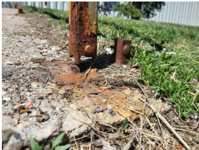
Photo #47: Corroded Railing - Entrance
