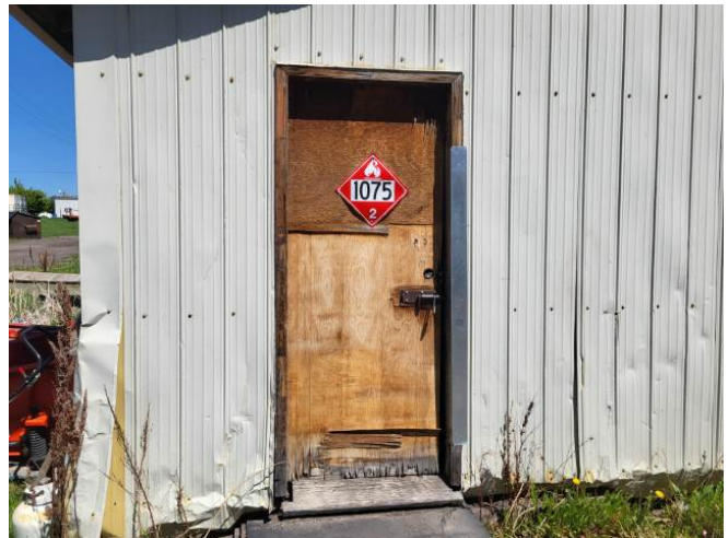
Storage Shed - Deteriorated Man Door
