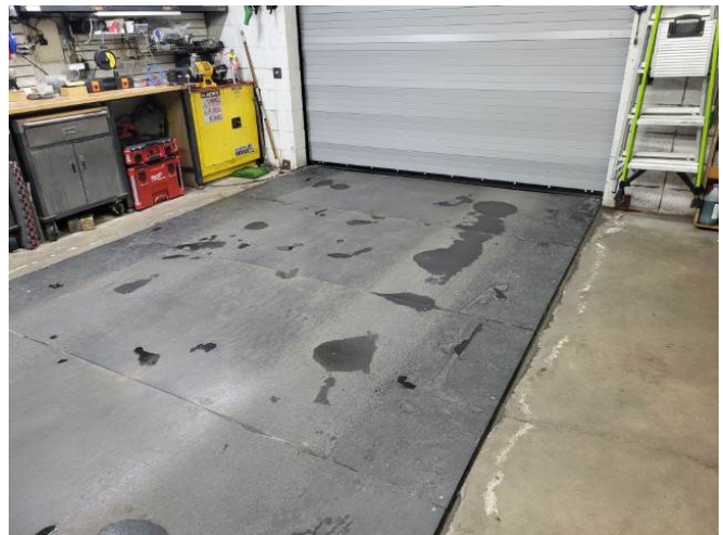
Zamboni Slab on Grade Covered with Rubber Panels (Small)
