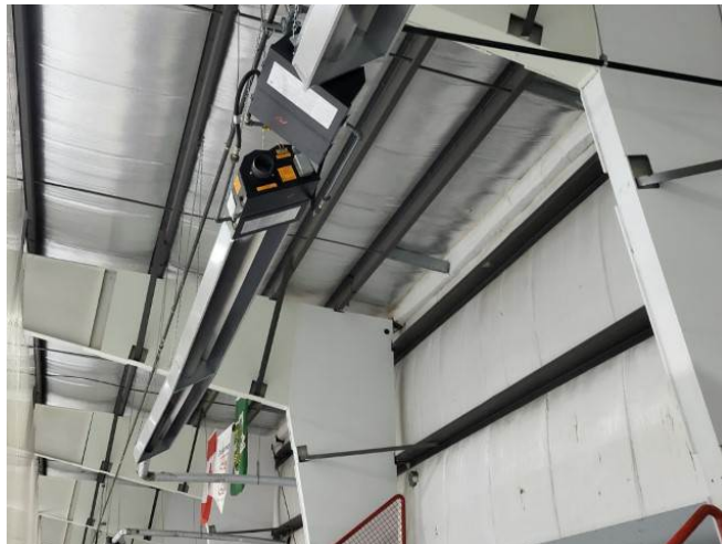
Photo #71: Suspended Infrared Heater
