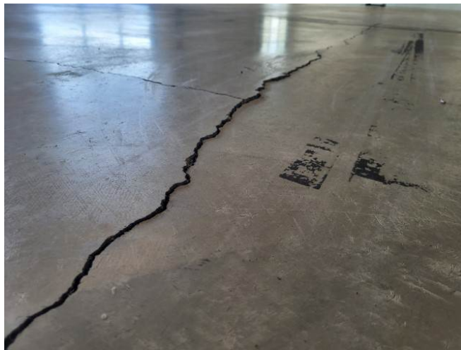
Photo #5: Cracking and Displacement in the 2nd Floor Slab of Undeveloped Area
