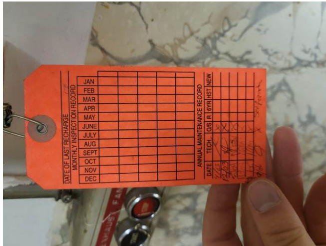
Photo #36: Chemical suppression System - Overdue
