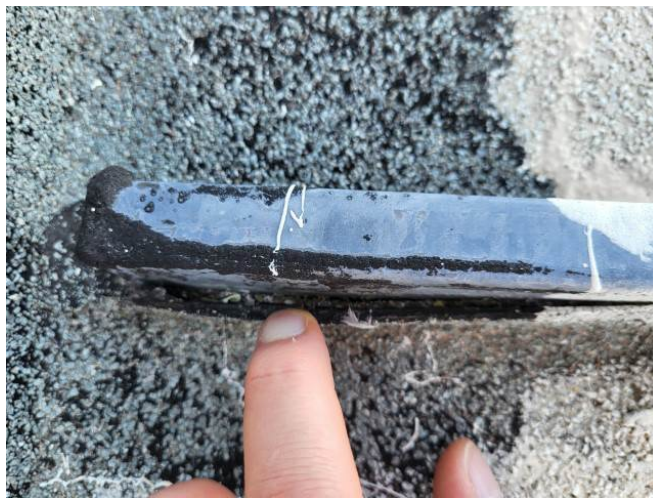
Photo #28: Debonded Roof Repairs Near Ribs
