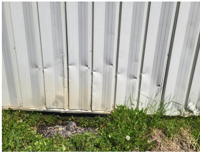
Photo #14: Dented Cladding - South Elevation
