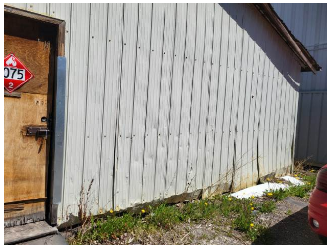
Storage Shed - Damaged Wall Metal Cladding
