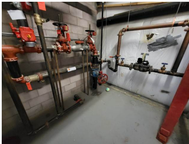
Photo #31: Sprinkler Risers
