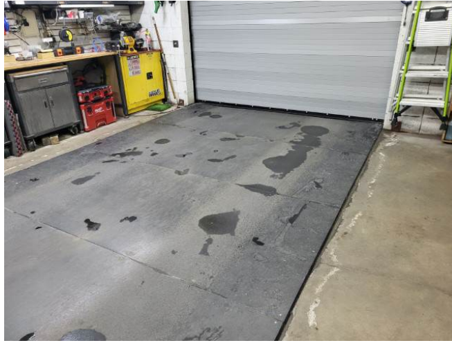
Photo #7: Zamboni Slab on Grade Covered with Rubber Panels (Small)
