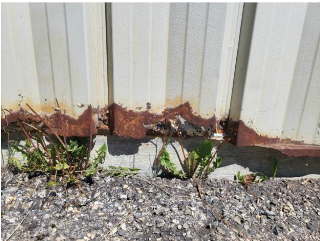
Corroded Metal Panel Cladding - South Elevation
