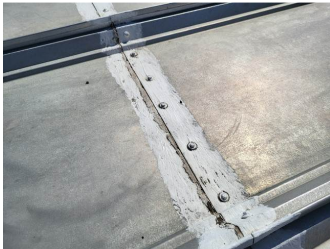
Photo #26: Deteriorated Roof Repairs - Fasteners
