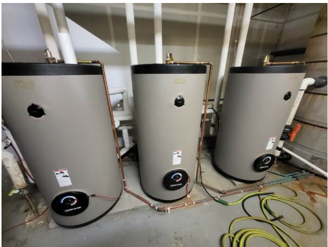
Domestic Hot Water Storage Tanks
