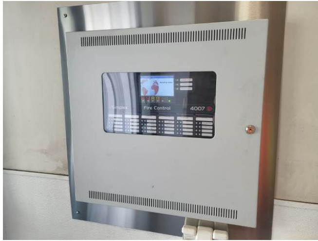
Photo #30: Fire Alarm Control Panel
