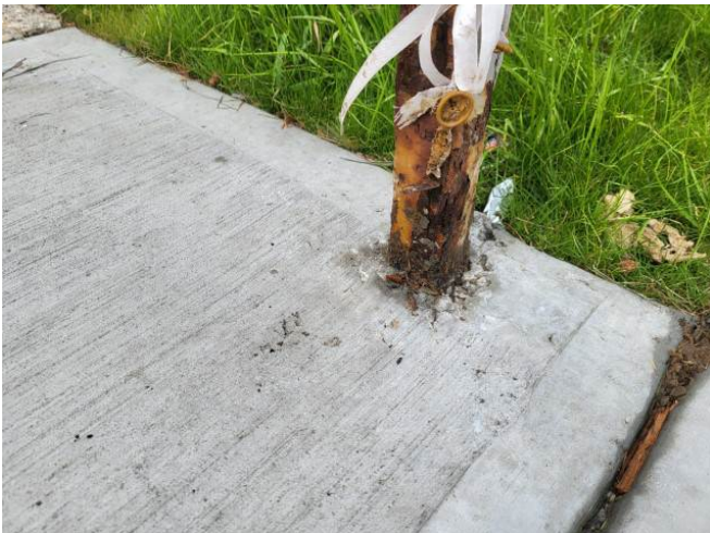
Aug 15_ Railing Embedded in Concrete_Corrosion Present
