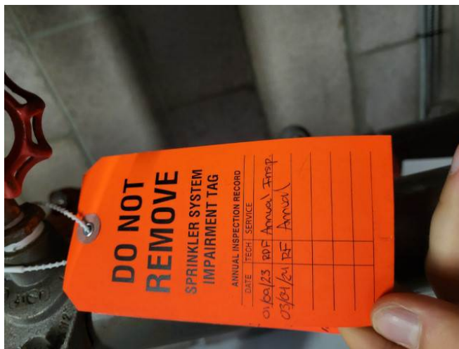
Photo #34: Sprinkler System - Overdue for Inspection
