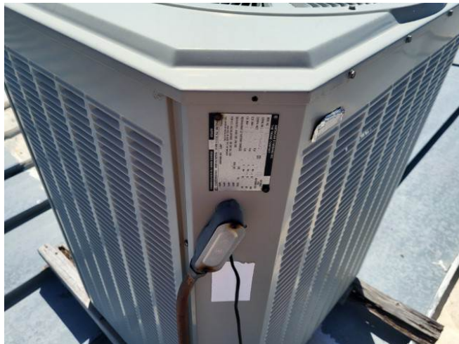
Photo #65: Condenser connected to Furnace
