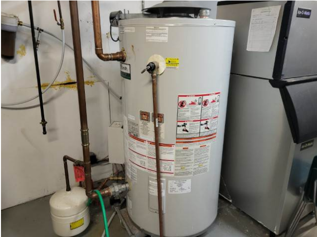
Domestic Hot Water Heater Serving Blue Arena
