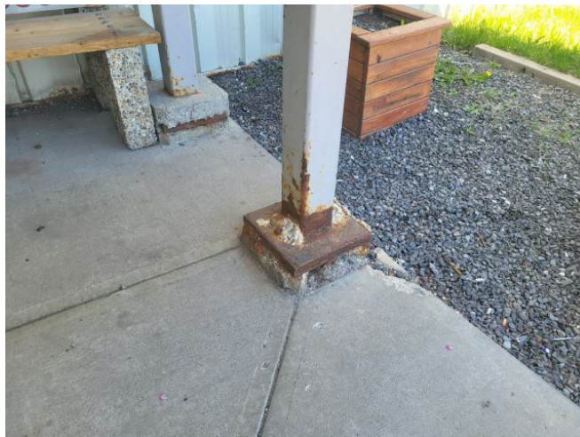
Photo #9: Corroded and Deteriorated Base of the Canopy Columns and the Columns Supports
