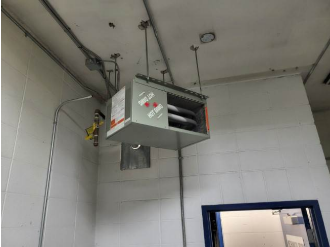
Natural Gas-Fired Suspended Unit Heater
