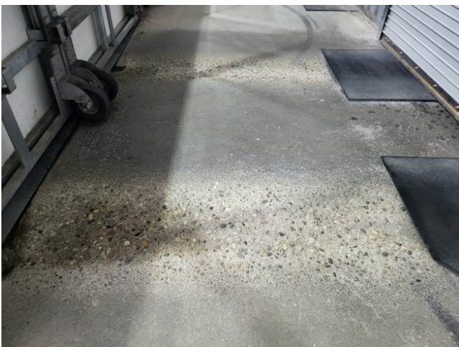
Deteriorated Slab on Grade in Zamboni Garage (Small)
