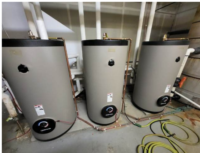
Photo #73: Domestic Hot Water Storage Tanks
