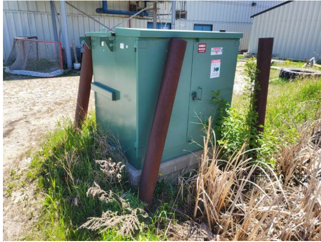
Photo #57: Pad Mounted Transformer - Tilted Bollards
