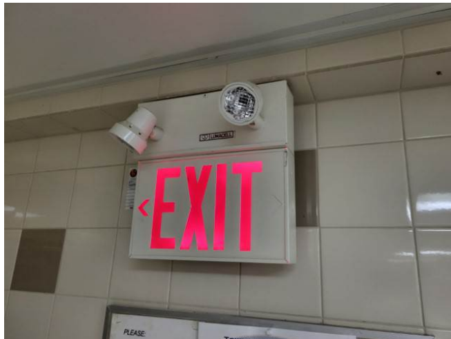
Photo #38: Typical Emergency Lighting and Exit Sign
