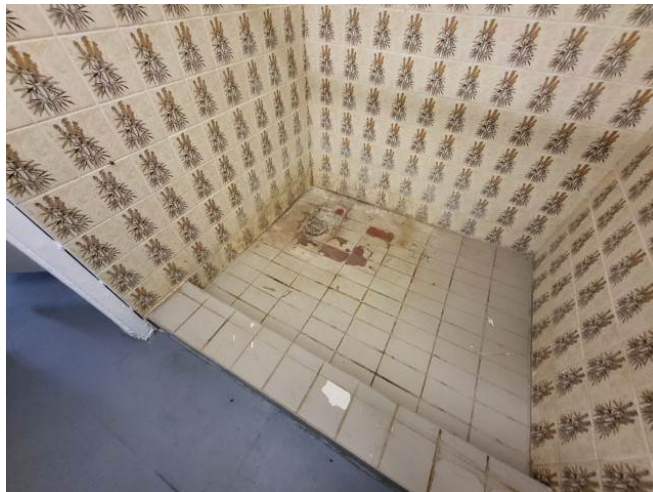
Photo #41: Cracked and Damaged Ceramic Tiles
