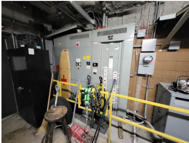
Photo #76: Main Electrical Service
