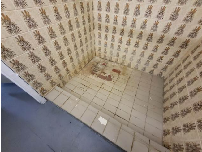
Cracked and Damaged Ceramic Tiles
