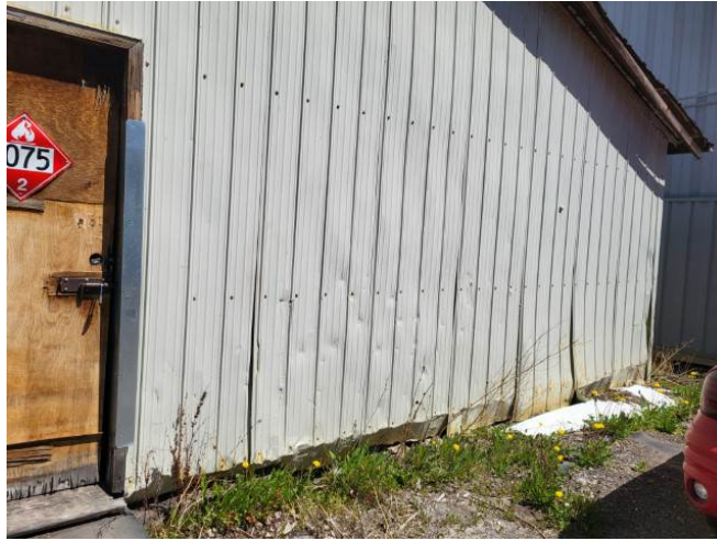
Photo #54: Storage Shed - Damaged Wall Metal Cladding
